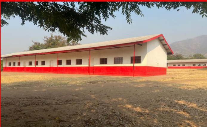
Rehabilitated school at EP Halima in Fizi health zone
