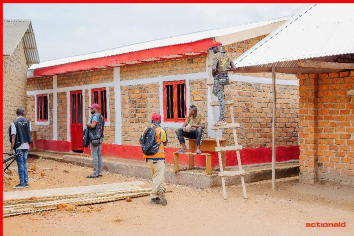
Ongoing construction at EP Ngunda in Koiyitanga community, Salamabila
